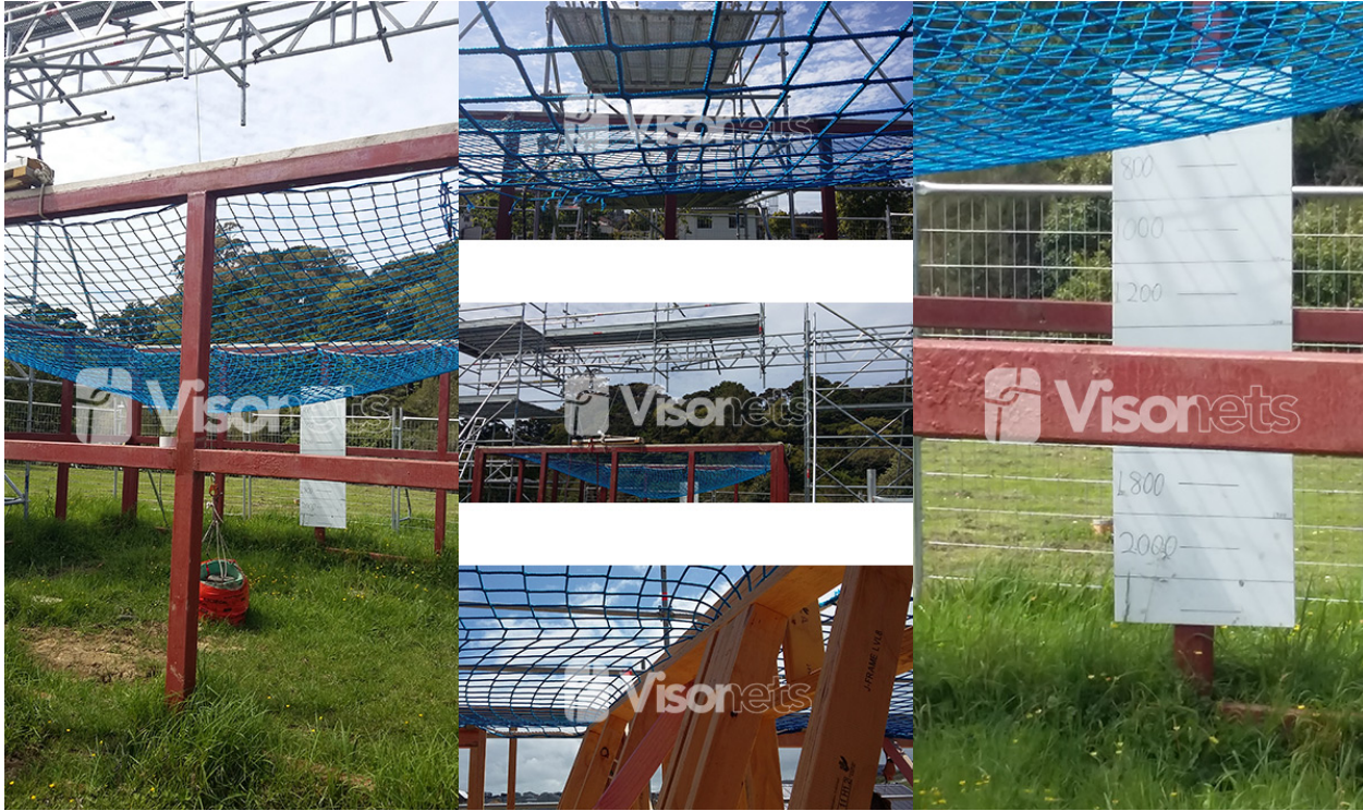
Safety net test facilities in New Zealand
